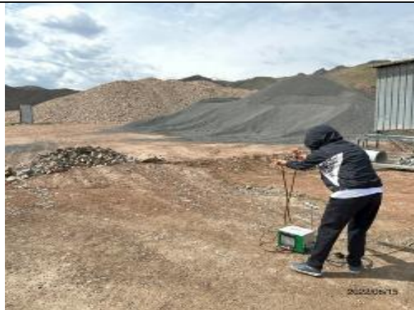
Photo 72. Air quality sampling at the Contractor’s rock crushing plant for Lot 2, km 81+200.
