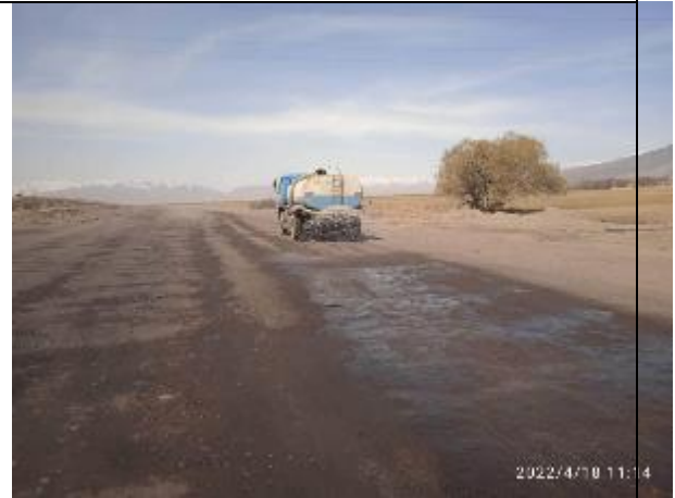
Photo 58. Watering along Lot 2 to control dust.
