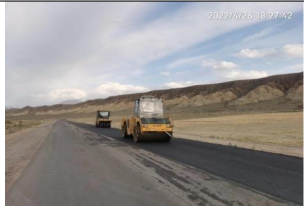
Photo 24 Binder course paving at km 74+120 - 75+00.
