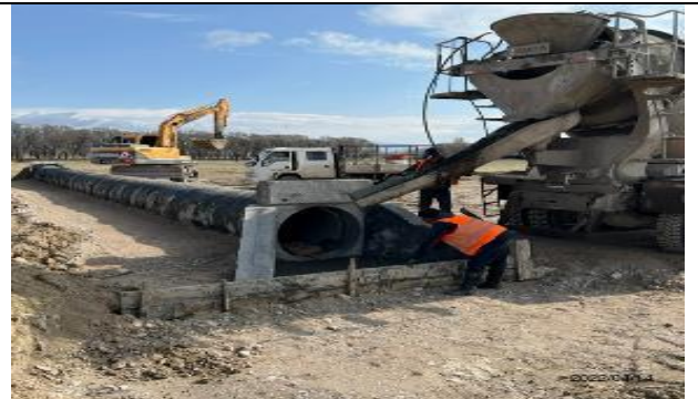
Photo 27. Construction of box culvert at km 62+700.
