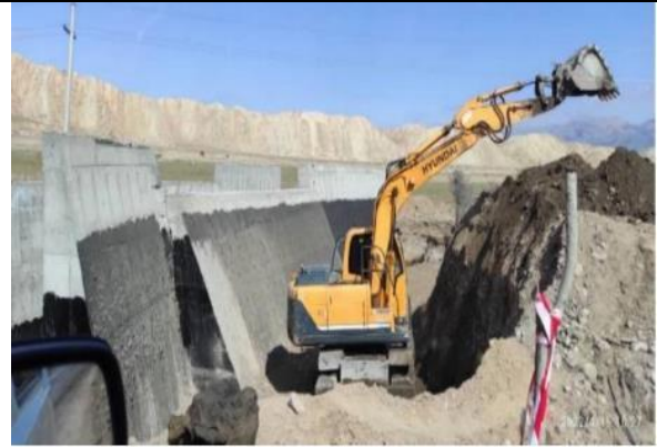
Photo 26. Backfilling of foundation and piers of Zharkurumdu River Bridge at km 88+795.
