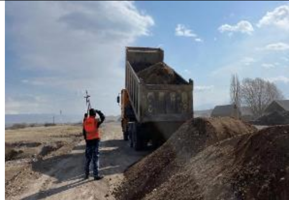
Photo 20. Subgrade backfilling at km 88+660 - km 88+740.
