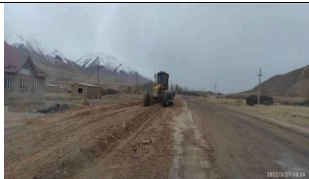
Photo 21. Construction of embankment at Km 89+340.
