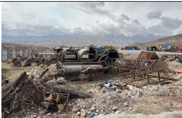
Photo 61 Scrap materials around the fabrication area.
