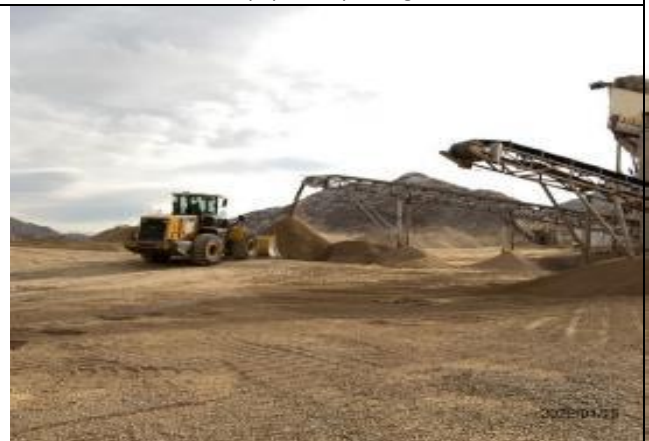
Photo 42. Lot 1 rock crushing plant.
