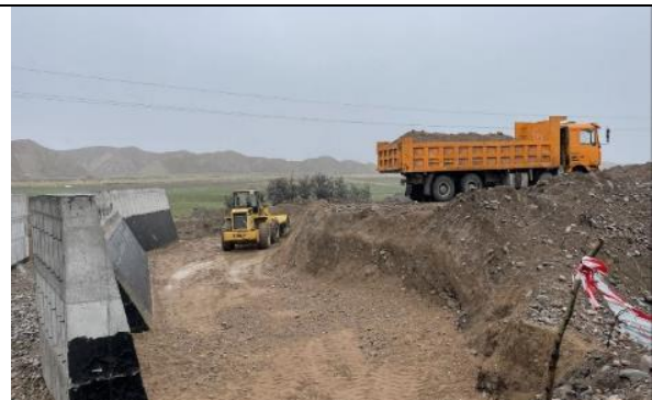
Photo 22. Backfilling of bridge at km 88+795.
