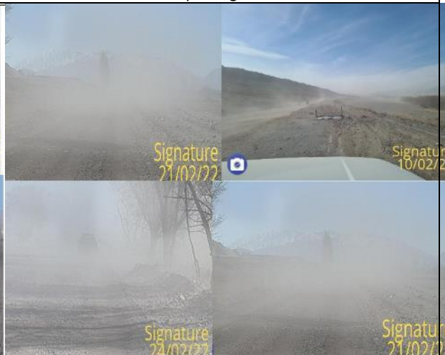
Photo 56: Dust at km 71+500, km 72+680, km 81 to km 86,
