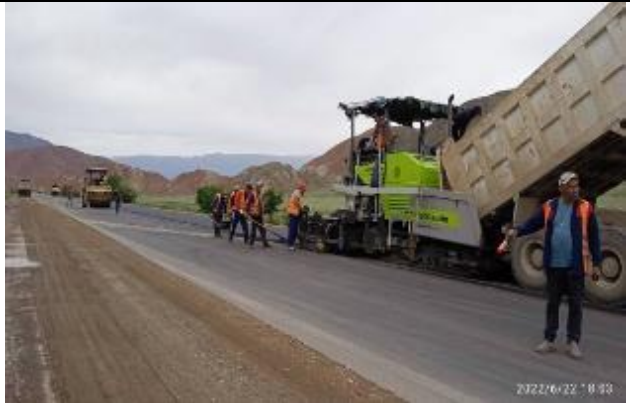
Photo 25. Binder course paving at km 17+564 - 18+677.
