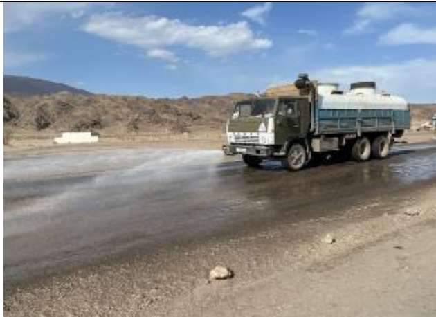
Photo 57. Watering along Lot 1 to control dust.
