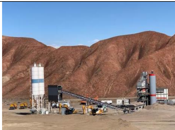
Photo 41. Lot 1 concrete and asphalt batching plants.
