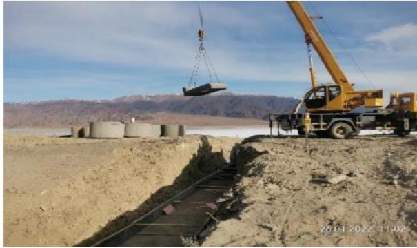
Photo 7. Installation of RCP at Km35+469.
