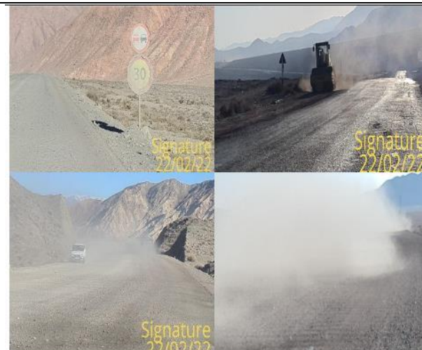
Photo 55: Dust at km 15+900, Km 41+750, km 16-36.
