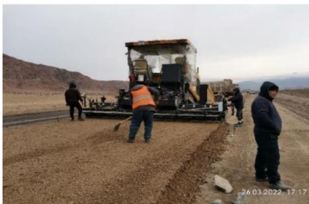
Photo 11. Base course construction at km16+300 – km 19+000.
