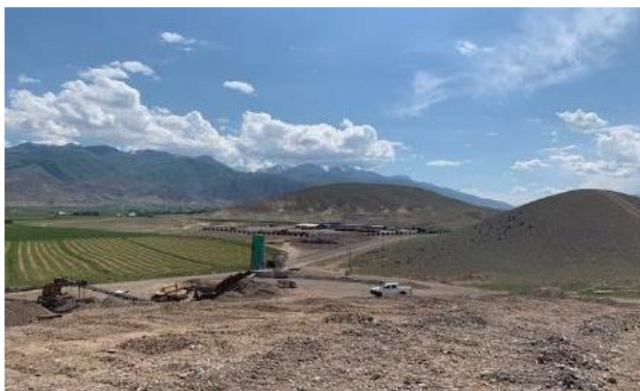
Lot 2 facility area with the rock crushing plant at the foreground and the Contractor's camp at background.
