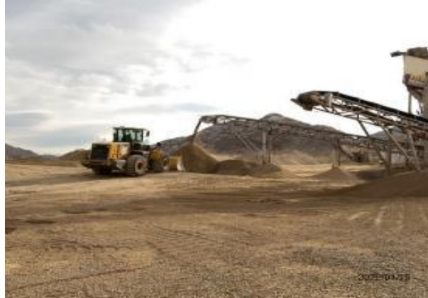
Photo 51. Rock crusher of Lot 1 in operation.
