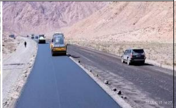
Photo 14. Compaction of binder course at Km15+600-km16+440 RS.
