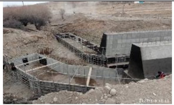
Photo 28. Installation of bridge retaining wall formwork for Ak-Uchuk River Bridge km 86+261.
