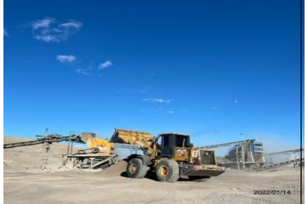
Photo 52. Rock crusher of Lot 2 in operation.
