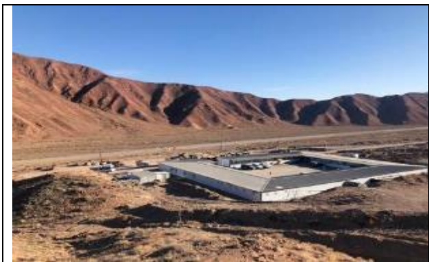
Photo 29. General view of Lot 1 campsite at km 16 + 100 (RS).
