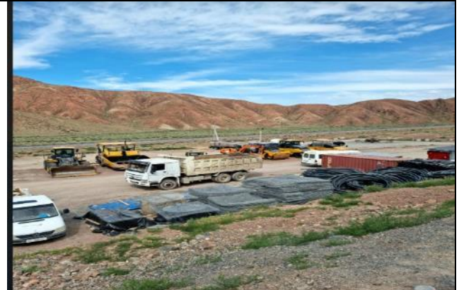
Photo 40. Vehicle and equipment parking area.
