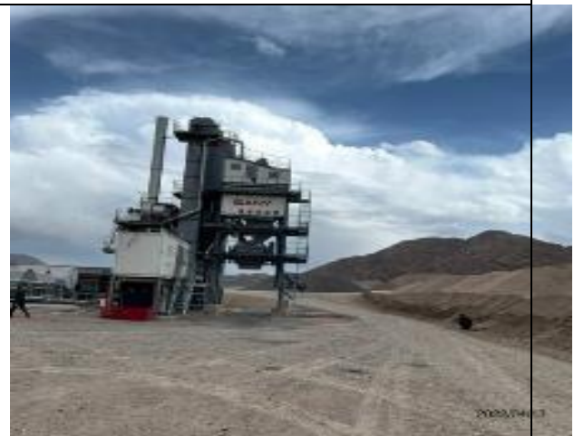
Photo 60. Asphalt plant in operation at Lot 1. Good facility and site maintenance.
