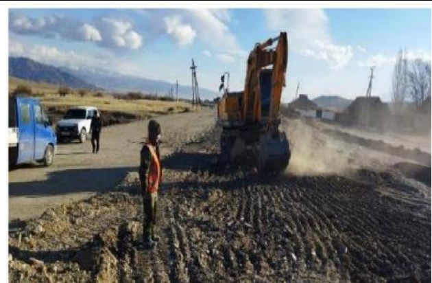
Photo 19. Existing a/c pavement being scarified at km 88+660 to km 88+750.
