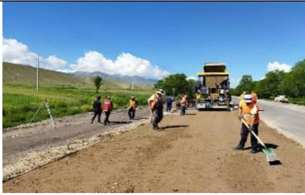
Photo 23. Crushed stone paving at km 83+000 to km 83+400 LS.
