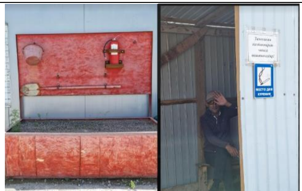
Photo 36. Left photo: provision for firefighting Right photo: smoking area.
