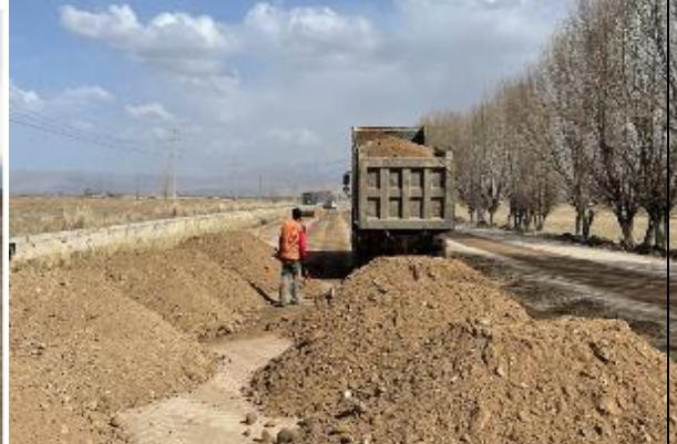
Photo 12. Filling of subbase at km66+740-km67+740 RS.
