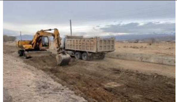
Photo 16. Grubbing works at Km 65 – km 300.
