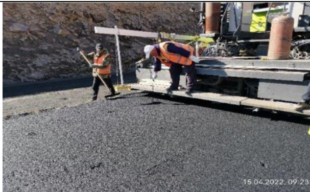
Photo 13. Laying of binder course at Km17+230 – Km17+500.
